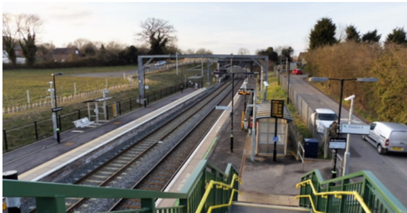
Fig 57. Alvechurch new rail station completed 2015
