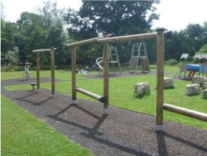
Fig 44. The new play equipment being installed at the Wiggin Field in 2015
